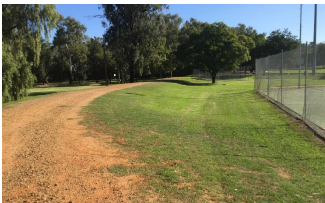
The existing levee bank south of Victoria Park Inner
