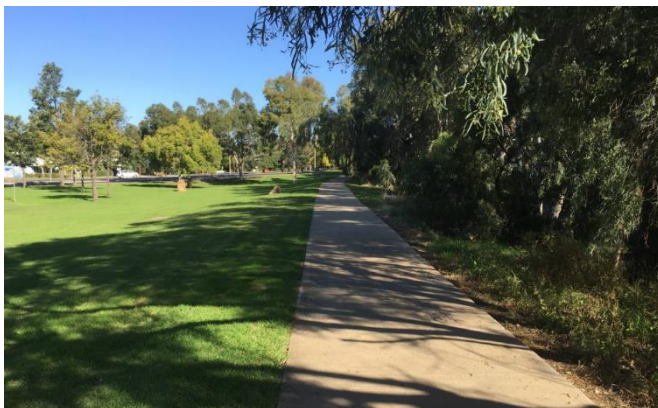
Existing levee bank – Udora Road
