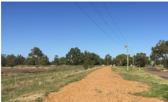
Existing levee bank – Udora Road
